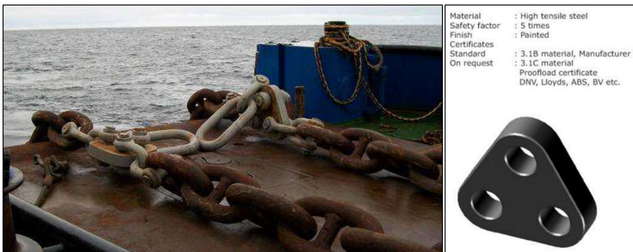
Figure 7: Triplates during mooring installation (left) and specification (right)
